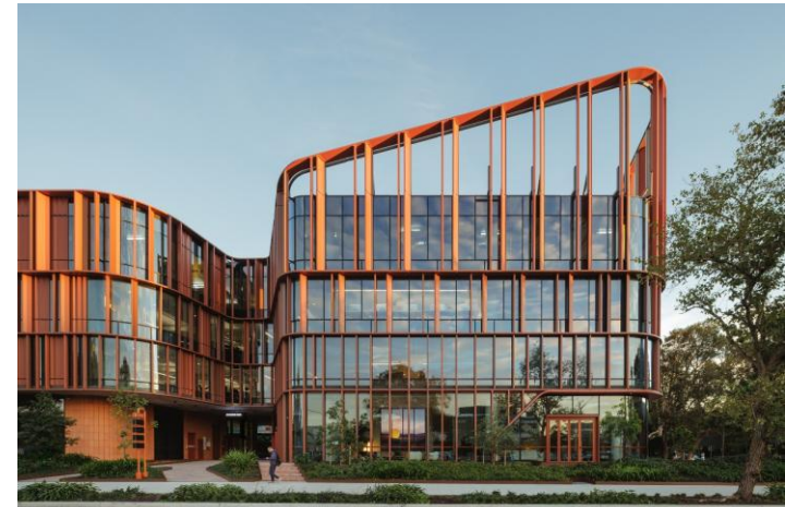
Pictured above is one the five assets that ACP II is providing private credit to, a campus-style Grade A office in Sydney, Australia
