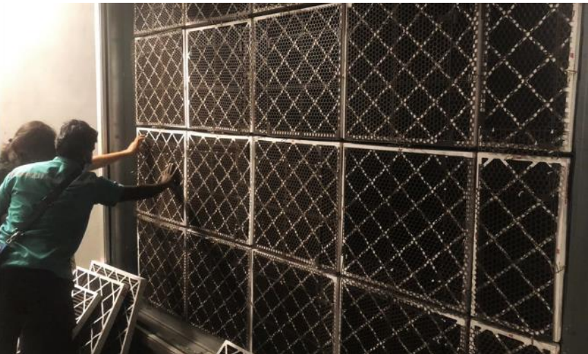
Installation of ceramic/polyethylene nets that acts as a natural ionizer generating a negative charge improving the function of heat exchanger, decreasing required cooling load, while also reducing air flow resistance faced by AHU fan at LogisTech
