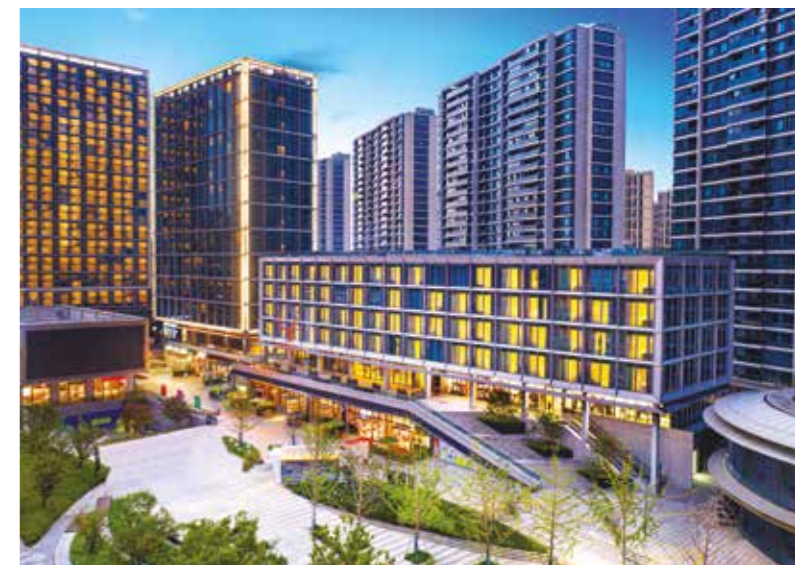
Ascott's first lyf-branded coliving property in China, lyf Mid-Town Hangzhou, opened in September 2021. It is located in the Gongshu district, near the Grand Canal, a popular UNESCO World Heritage site noted for its historical relics.
