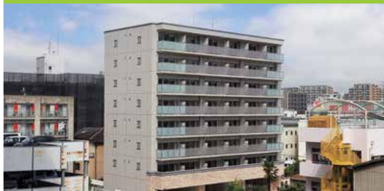
▲ A multifamily property, which is part of the six multifamily assets in Central Osaka, Japan acquired by COREF.
